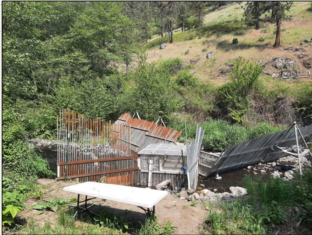
Six Mile Creek Weir (Photo by Mike Kosinski)
